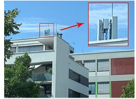
5G 3.5 GHz Cell Site of Deutsche Telekom in Darmstadt, Germany
