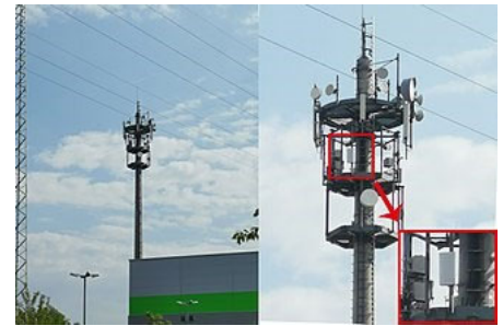
5G 3.5 GHz Cell Site of Vodafone in Karlsruhe, Germany
